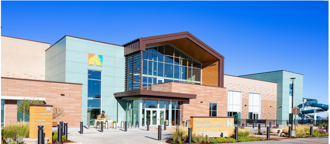
DETAIL: NORTHGLENN RECREATION CENTER, SENIOR CENTER AND THEATRE, NORTHGLENN COLORADO, / BARKER RINKER SEACAT ARCHITECTURE
