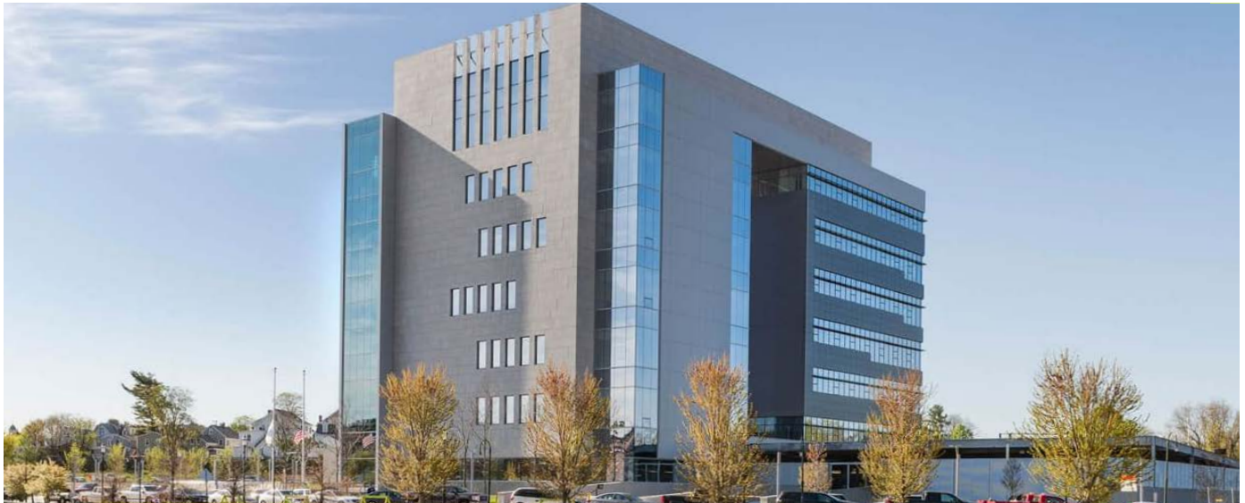
ELEVATION: LOWELL JUSTICE CENTER / FINEGOLD ALEXANDER ARCHITECTS | PHOTO CREDITS: ANTON GRASSL
