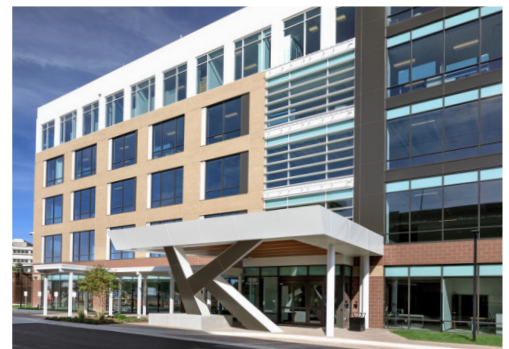
DETAIL: ACM PANEL CLADDING AT SOFFIT
