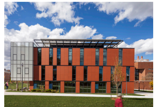
DETAIL: EXTERIOR TERRACOTTA PANEL FACADE
