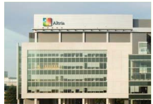
DETAIL: ACM CLADDING
