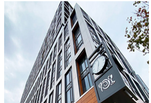
DETAIL: VERTICALLY-ORIENTED UHPC (FIBER CONCRETE) PANELS
