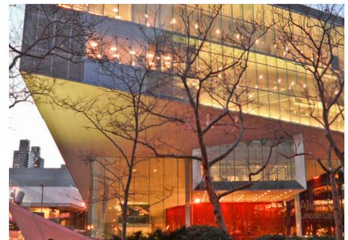
DETAIL: SWEEPING FIBER CEMENT SOFFIT
