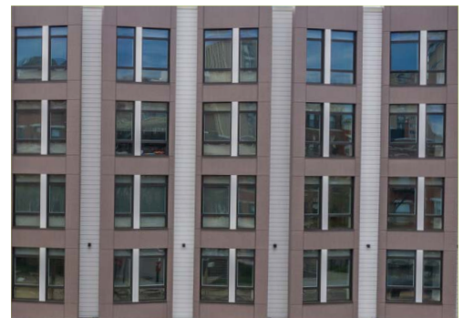
DETAIL: SWISSPEARL FIBER CEMENT PANELS
