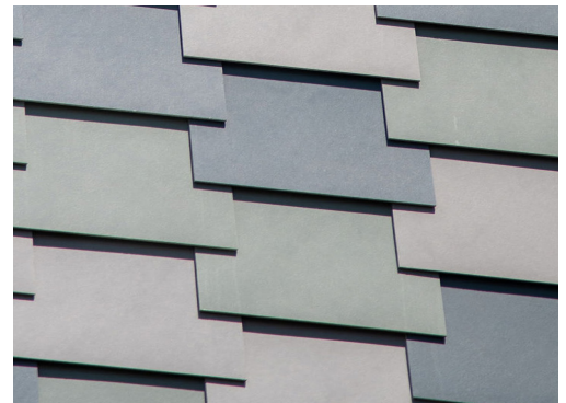
DETAIL: LARGE FORMAT FIBER CEMENT SHINGLES
