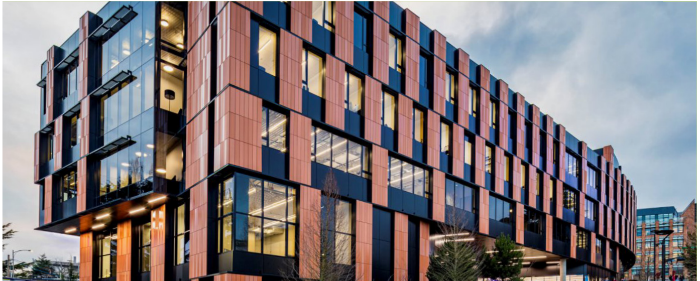
ELEVATION: U OF WASHINGTON PAUL G. ALLEN SCHOOL OF COMPUTER SCIENCE & ENGINEERING / LMN ARCHITECTS
