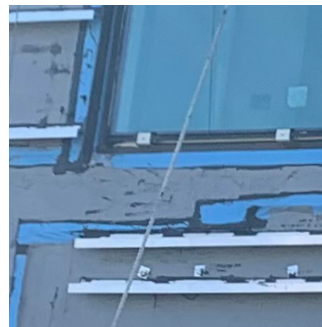
PHOTO: EXCESSIVE USE OF SILICON SEALANT WHEN Z GIRT IS APPLIED TO THE WALL
