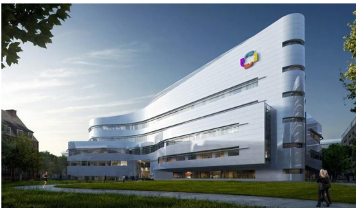
Harford Hospital Medical Office Building (Hartford, CT) Perkins + Will / ACM
